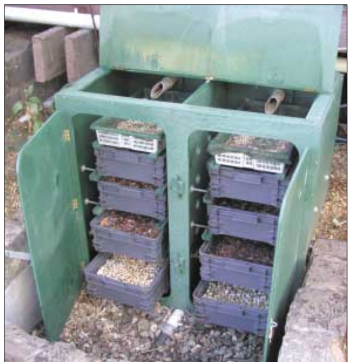
The CERES designed bio-filter captures and treats the wastewater that comes from the cafe.
